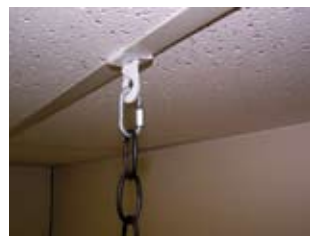
Lift unit onto 1 ceiling clip.
