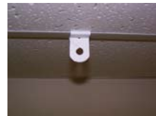
Clip properly installed.
